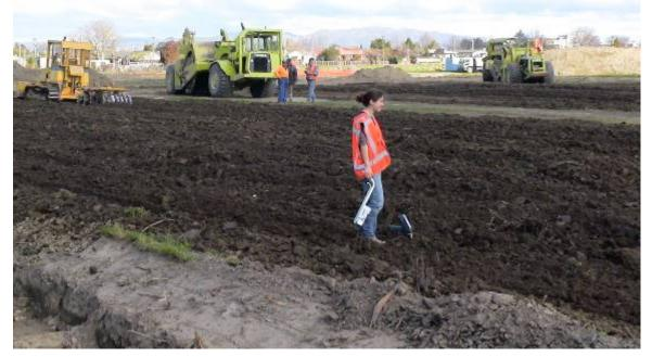
Validation with XRF of disked layer in progress. Temporary mix-pad in the background.
