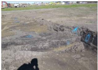
Here As contamination removed to a depth of 0.7 m
